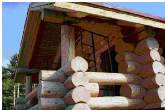
Fig. 3.10. The end wood blocks of logs (source Kon Corporation, http://www.dom.kon.ru/ )
